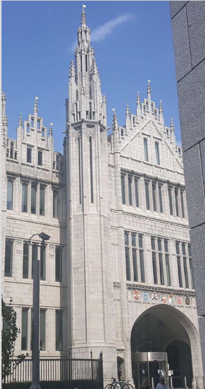
Marischal College The early 20th century front elevation uses the finest Kemnay ashlar-cut blockwork and detailing
