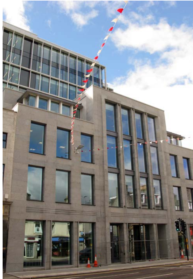
The Silver Fin The frontage faces onto Union Street, the use of light-grey granite cladding respects the street's granite heritage and colour, whilst the use of glazing in the taller element behind helps to reduce its massing
