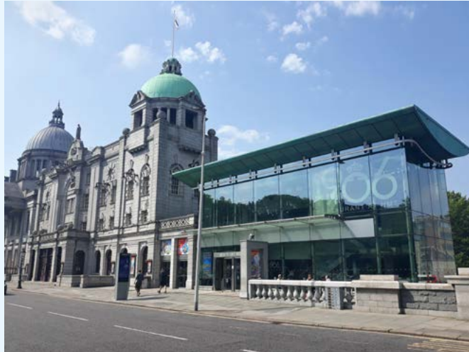
The green-tinted glass extension to His Majesty's Theatre reflects the colour of the building's copper dome above
