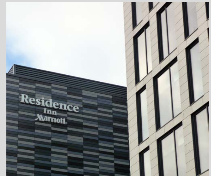
Imported granite cladding panels have been used on new buildings in Aberdeen such as Marischal Square
