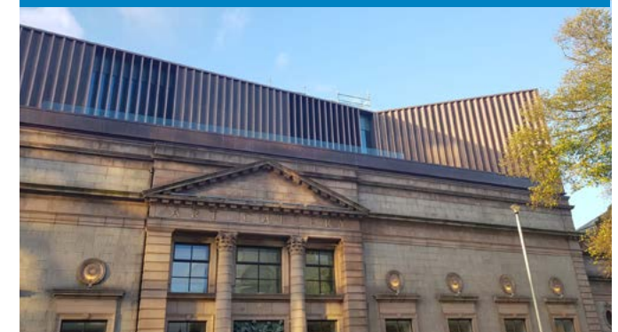
Aberdeen Art Gallery The contemporary roof extension to the Category 'A' listed Aberdeen Art Gallery has been designed as an honest, clearly modern addition to the original building and its granite façade below. The use of pink/brown copper cladding serves as a good match for the pink Corrennie granite used in the façade embellishments
