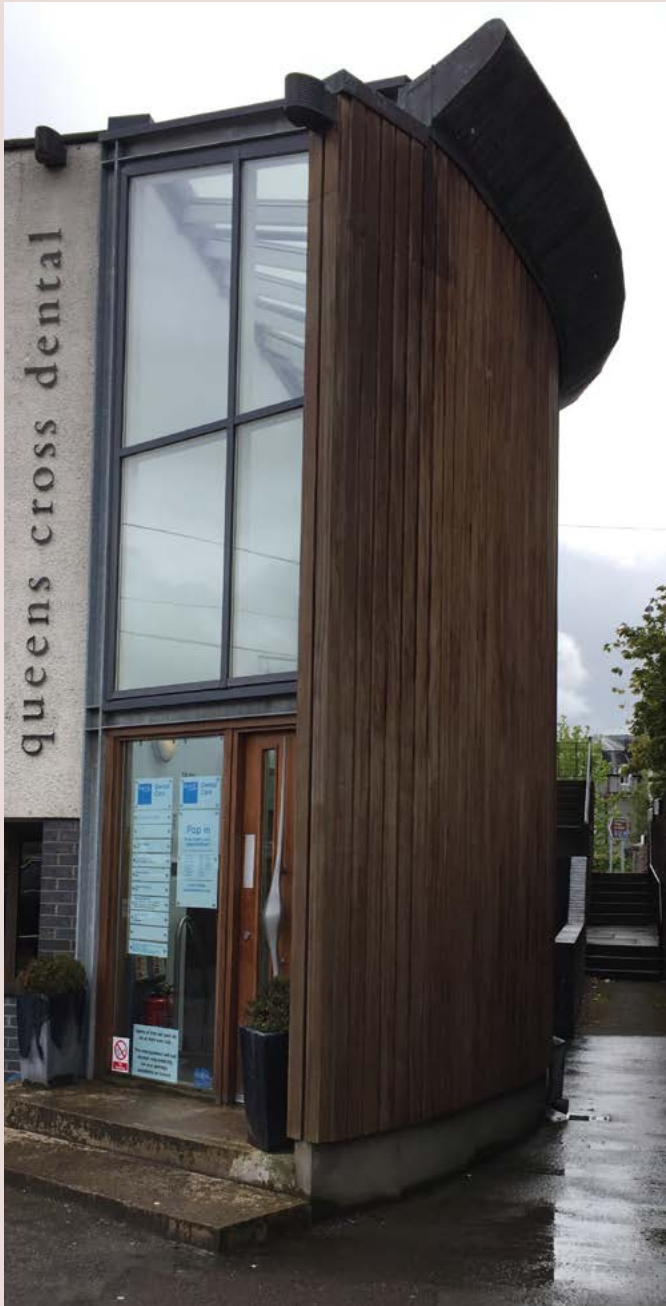
Vertical timber cladding to rear extension of Queen's Cross Dental in interesting curve design
