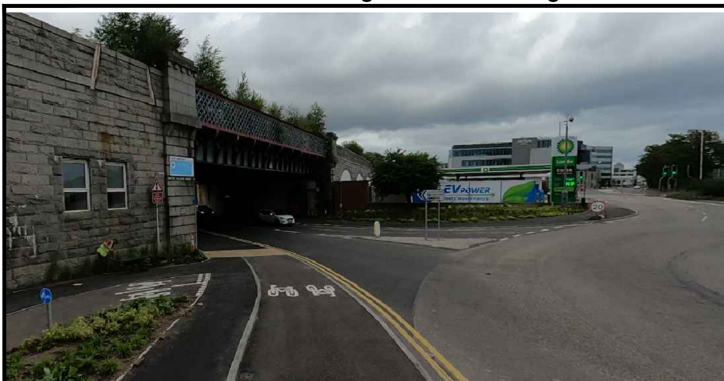
B - Uncontrolled Crossing over QEII Bridge
