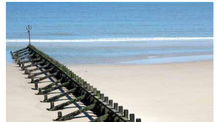
Image of the Groyne structures which are positioned along Aberdeen Beach
