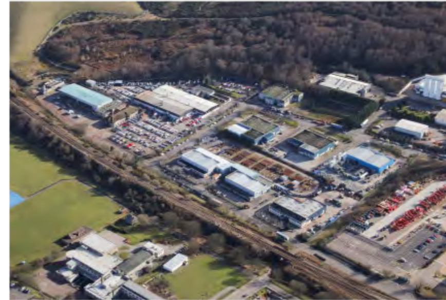
East Tullos Industrial Estate
