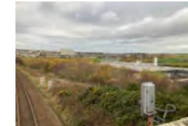
Railway Crossing (to be closed)
